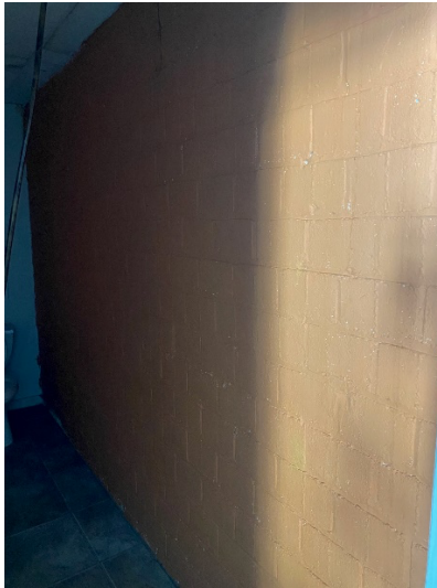
Figure 2. XRF Readings 1231 & 1232, on the block wall inside the bathroom of the Deacon School, were found to have lead readings of 1.0 \text{ mg/cm}^2
