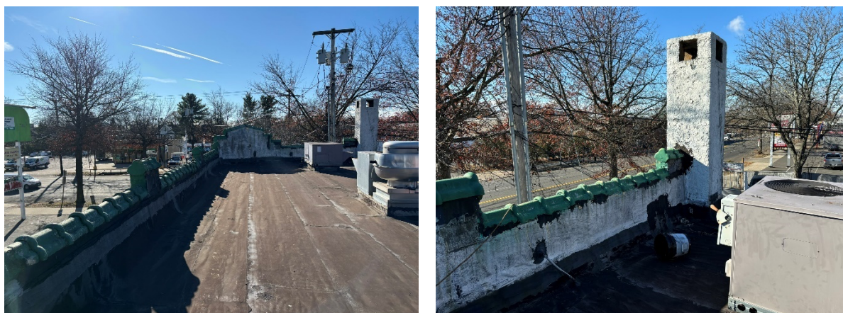
Figure 3. XRF Readings 12304 to 1306, on the roof (green paint on parapet), were found to have lead readings of 6.3 \text{ mg/cm}^2 to 10.7 \text{ mg/cm}^2
